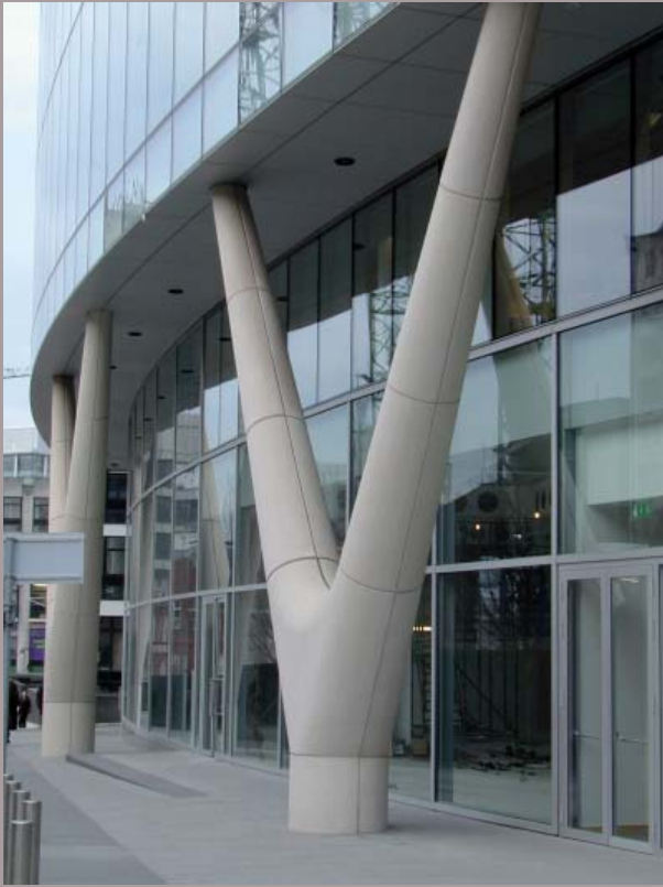
Bespoke Column Casings No 1 Spinningfields Manchester
