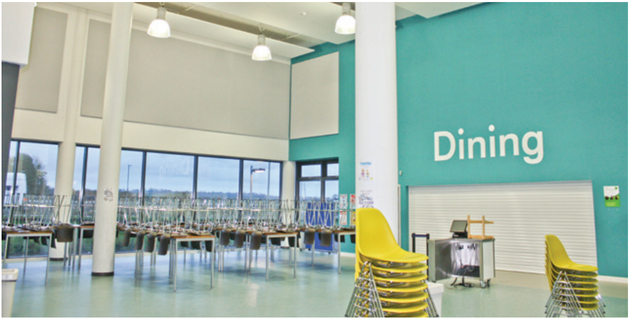
WALLSORBA® Type C panels installed in school Dining Hall
