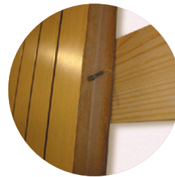
Screw fixing
