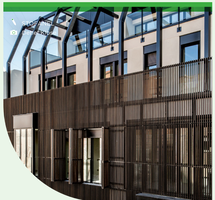
Alfonso X residential building - ASPRIMA-SIMA Award (5100 m 2 ) Madrid, Spain
